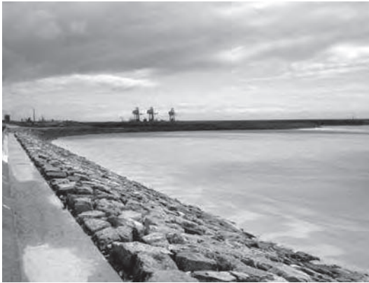
Figure CS12.3 Rock armour fronting promenade seawall
