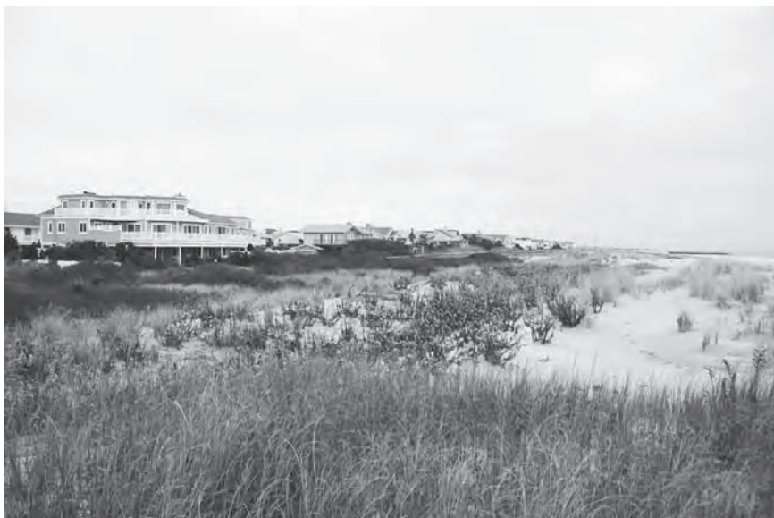
Figure CS7.3 The dune created in 1987 in the southern portion of the improved beach, showing the foredune crest on the right created by sand fences and the species diversity on the left resulting from protection by the high crest
