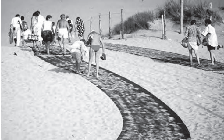
Figure 3.1 Fencing and rubberized access mat of beach/dune areas on the western coast of France
