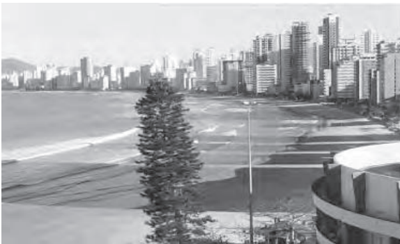
Figure CS8.4 Among the most significant problems regarding Praia Central in Balneário Camboriú is shadowing caused by seashore buildings, responsible for the desire for beach enlargement
