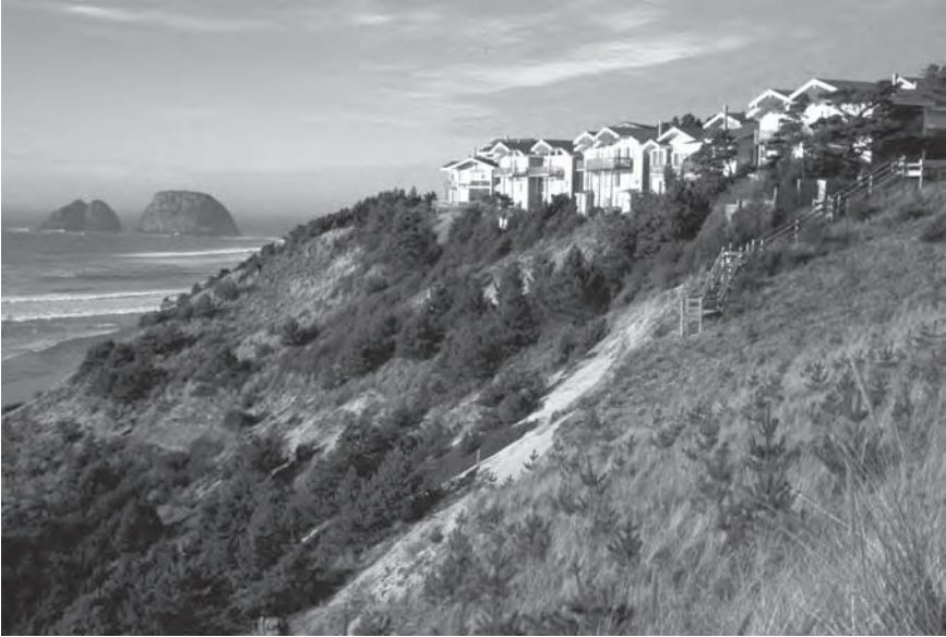
Figure CS9.4 The front line of condominiums of The Capes development, lining the edge of an old landslide
