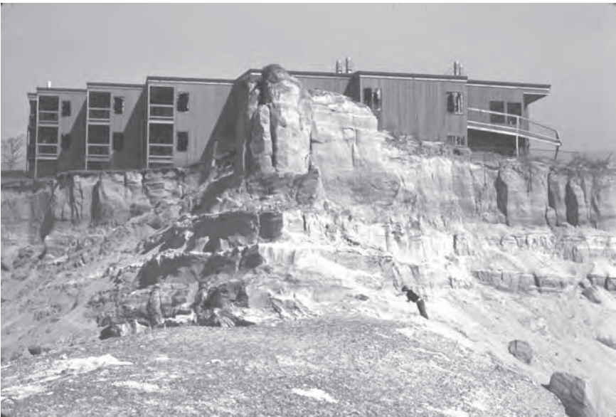
Figure CS9.2 The initial stages in the destruction of condominiums built in the Jump-Off Joe area of Newport
