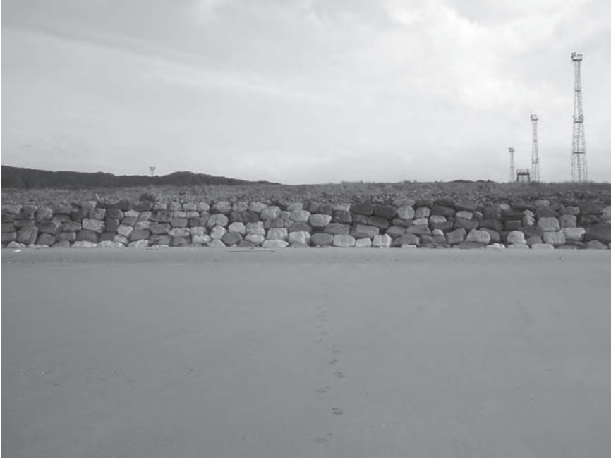
Figure CS12.6 Slag and rock armour revetment
