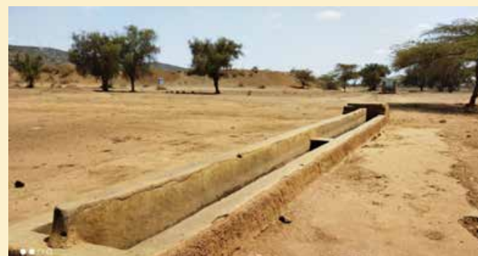
Water trough at Marandagwa, Kajiado
