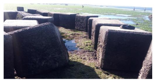
Plate 4.8: Massive blocks at Vasco da Gama Pillar
