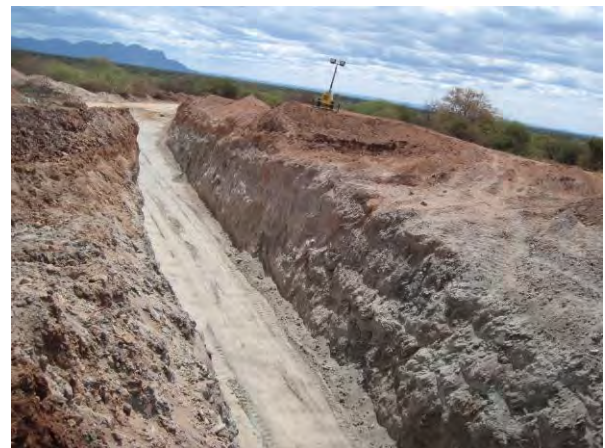
Figure 5 Access road into the pit
