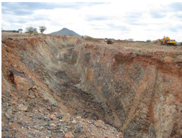
Figure 3 Excavation of a pit, development method
