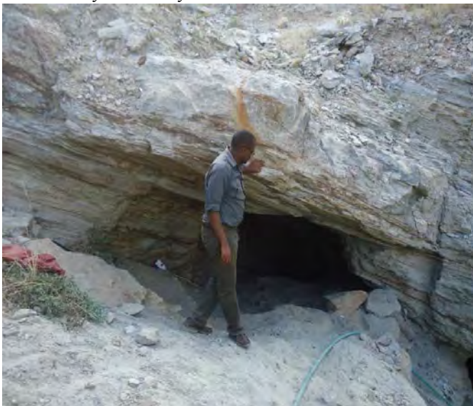
Figure 5: Tunnels cut and left open posing danger to people
